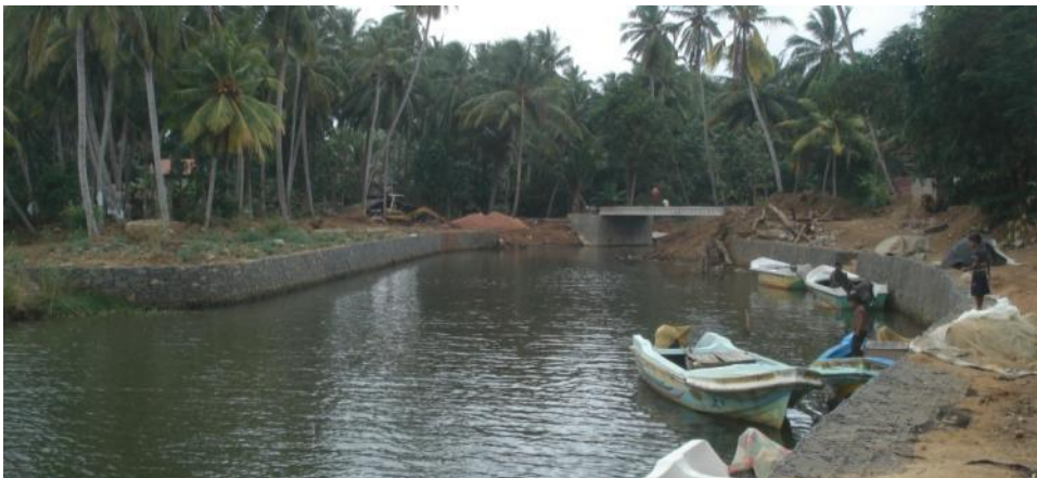
Figure 5 A new bridge under construction
