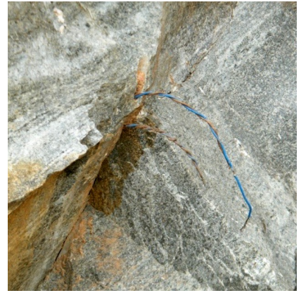
The rock blasting taking place is a threat to soil stability and a disturbance to the fauna
