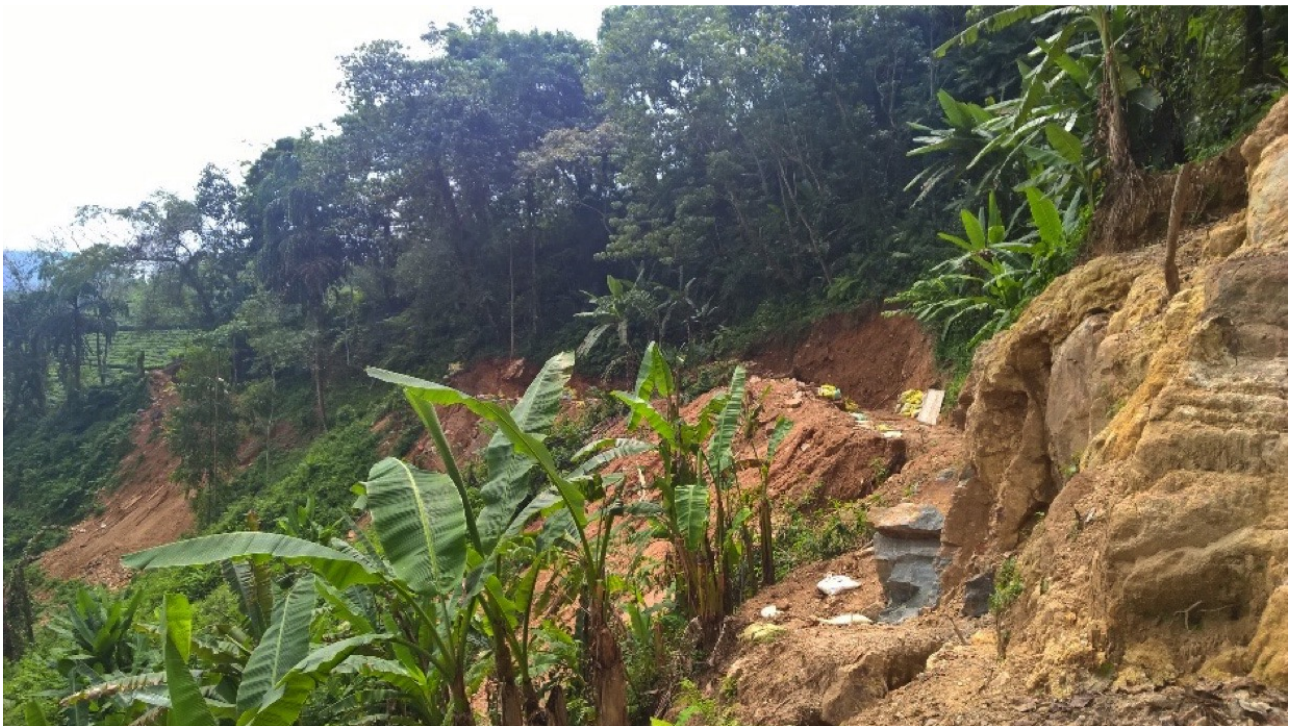
Part of the penstock has been cut along a slope, increasing risk of earth slips
