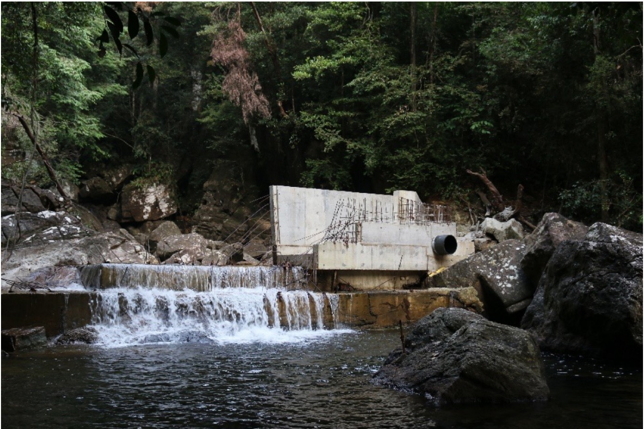
The incomplete weir
