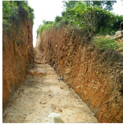
Tea lands on higher elevation have been cut through to construct the penstock
